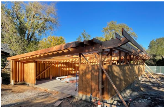
View from SW Corner: 11/3/21
