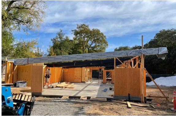
Roof Glulam Beams: 10/19/21 Each beam weighs over 1850 lbs
