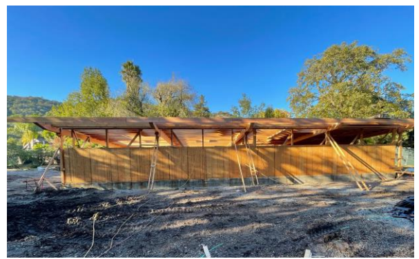
South Face of Facility: 11/3/21
