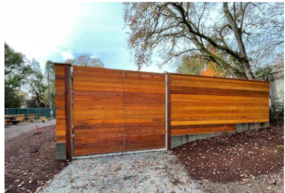
East Entrance Dual Swing Gates
