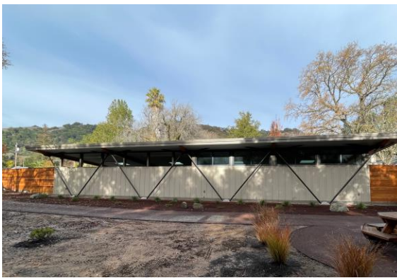
Maintenance Facility South Face (Front)
